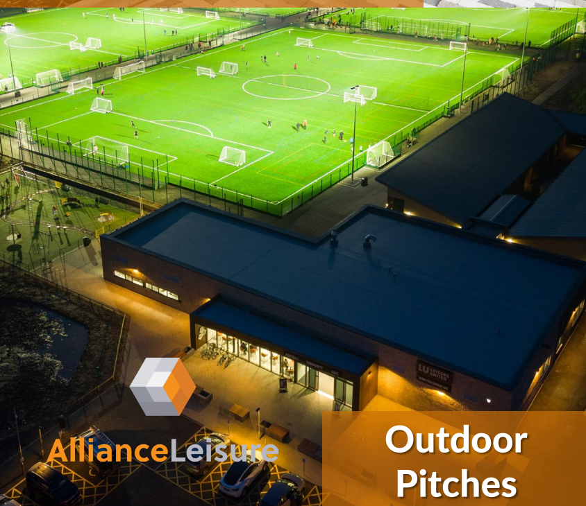
New Build of Sport & Leisure Facilities
